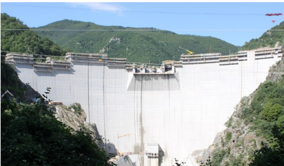
Tsankov Kamak Dam
