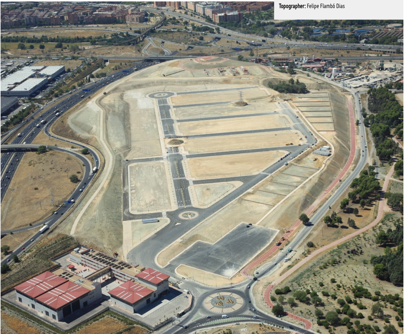
Aerial view of the enlargement
